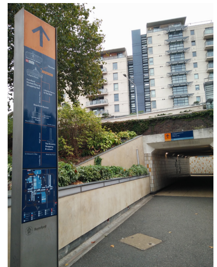
O4 – Romford Roundabout underpass
