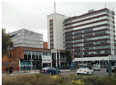
02 – North House – 11 storeys
